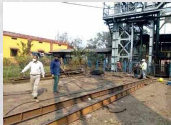
Figure 2. Photographs of the optical fiber bundles embedded in HDPE pipes being spliced together in the laboratory (left), and the fiber cables being lowered through the mine shaft to the pit-bottom at Jhanjra underground coal mine (right).
