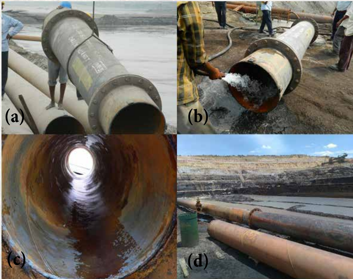
Fig. 3 Phase-II field trial : (a) Pipe-II taken out from mainline for inspection (b) Pipe-II is being washed and cleared of debris (c) the coating was found intact (d) Pipe-II is being deployed back to the mainline
