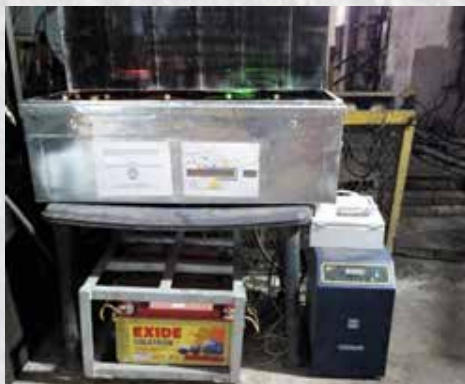
Figure 3. Photographs of the solar-powered artificial light coupling system installed at Jhanjra coal mine (left). The lasers and the optical coupler assembly used for illumination are shown (right).
